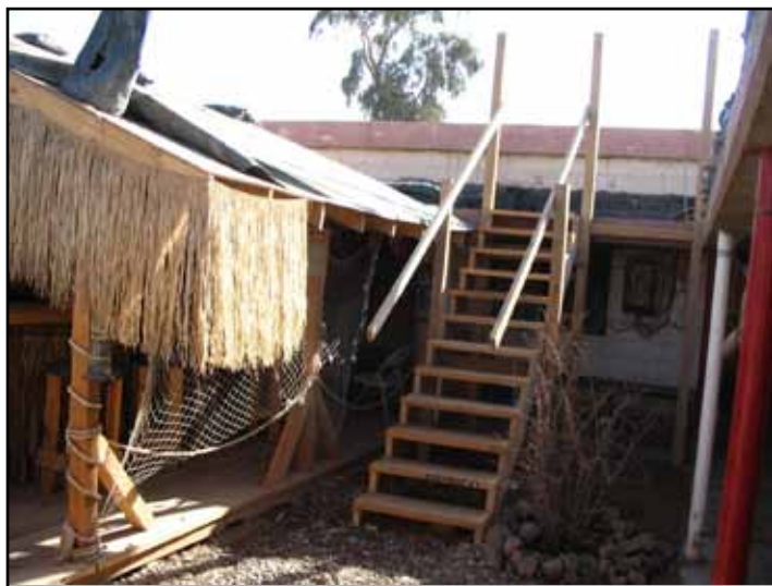
The stairs to the upper deck. A railing was added to complete Col. Lovejoy's safety requirements just hours before the New Years Eve Party.
